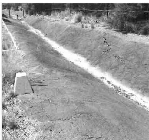
Figure 13: Existing Asphalt Perimeter Drain
