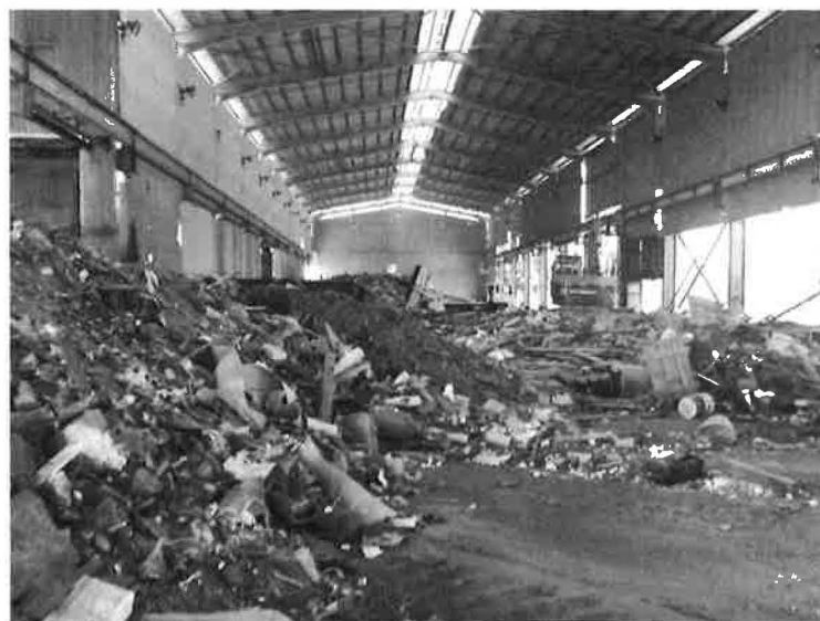
Figure 9: Existing Waste Stockpiles within the Main Processing Building
